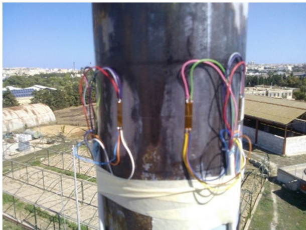
Fig. 21 Strain gauges installed and wired on the top mast of the tower
