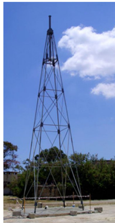
Fig. 3 The supporting lattice tower
