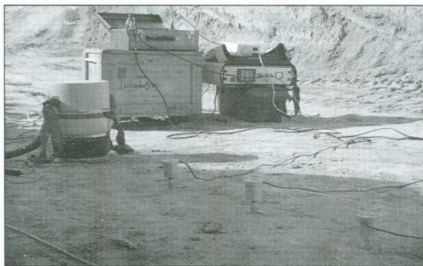
Figure 1: Continuous Surface Wave System being used on a sandy subgrade at the south of Iran (Maroon).
