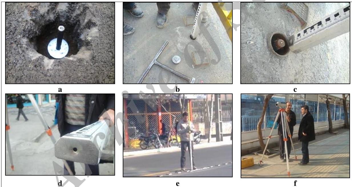
Figure 8. Steps of the installation of measuring equipments and ground settlement leveling
