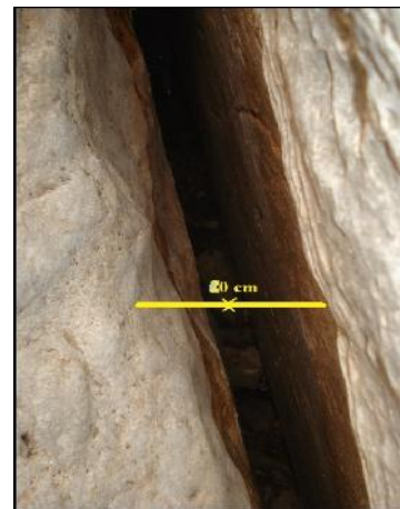
Figure 6. A major opening created by fault at the beginning of gallery No. 1
