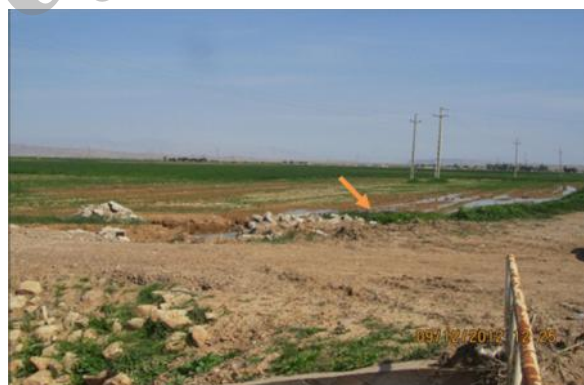
Figure 8. A view of drainage area covered by the irrigation system of Dasht-e Abbas
