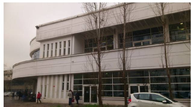
Fig. 2 View of north façade of the building
