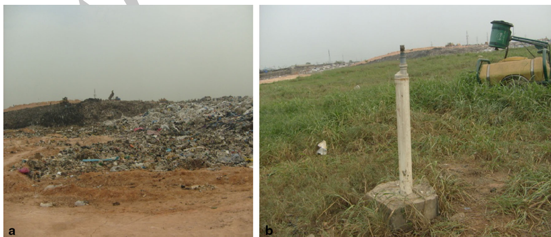
Fig. 4 Portions of the Olusosun landfill (a partially capped areas; b a well-head for LFG capture)
