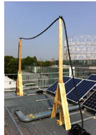
Fig. 5 Built structure for simulating medium voltage overhead lines shading
