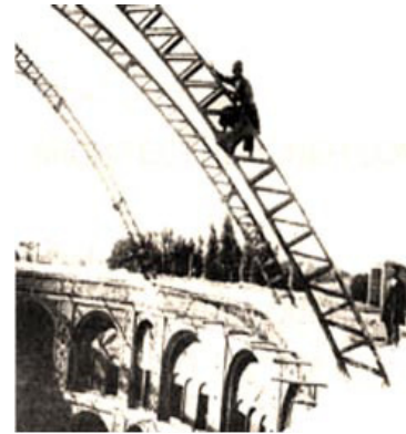
Fig. 12. Renovation of Dolat Masque ceiling using metal structures (Source: http://www.vista.ir/?view=context&id=296133 )
