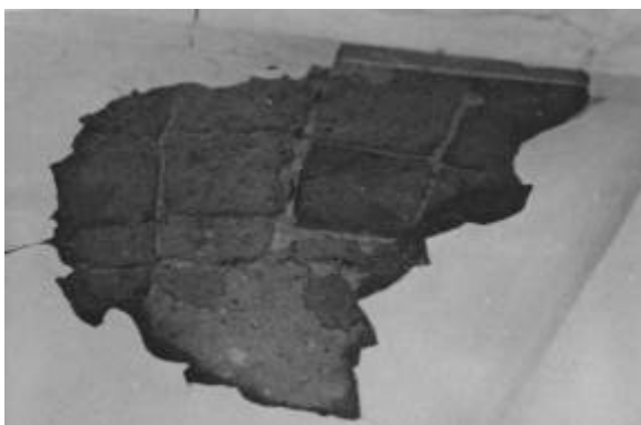
Fig. 7, 8. Construction details of the Lapoosh vault and a Plentiful vault showing the brick binding, The House of Attars, Kashan
