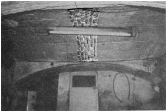
Fig. 4, 5. In Kashan and Tehran , houses the belts are clearly evident in the Lapoosh vaults (Source: The document centre archive of the architecture faculty of Shahid Beheshti University and the paper "Above the Geometry of Vault and Dome").
