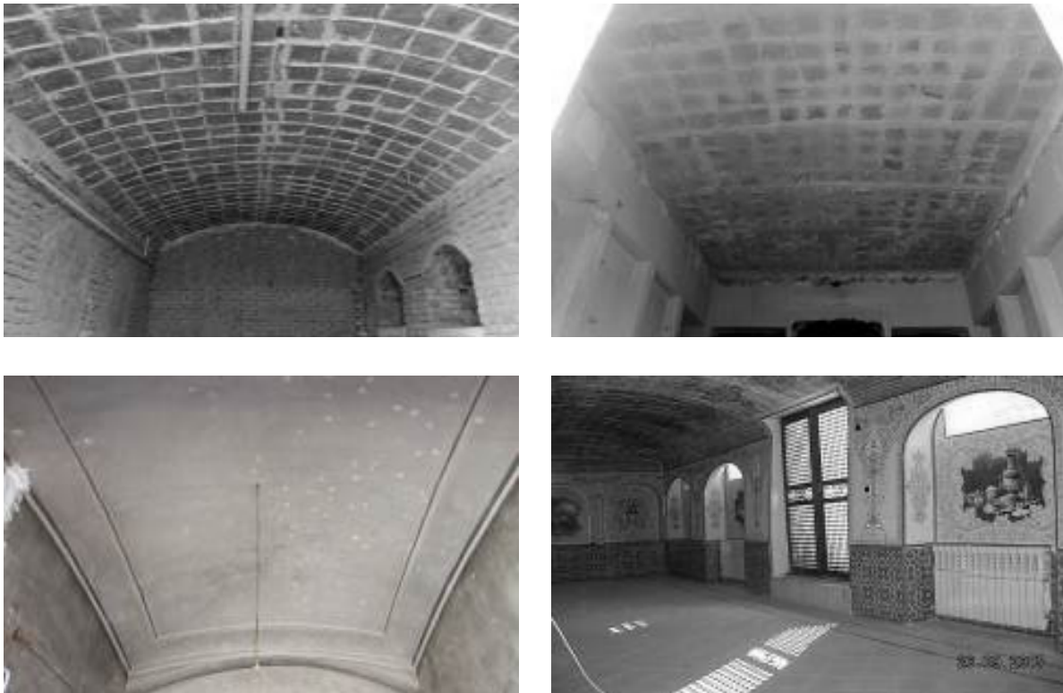
Fig. 16. A few Qomi-poosh vault samples with different deflection (Source: architect Helli's personal archive).
