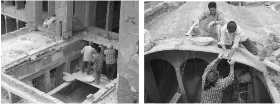
Fig. 14. The stages of building the Qomi-poosh vault (Source: architect Helli's personal archive).
