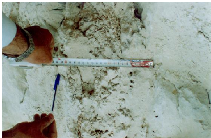
Figure 1. Fault thickness in Kangir Dam, Iran.
