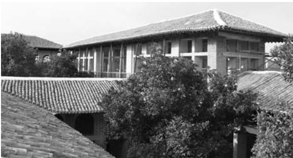
Fig. 7: A view of courtyards and building B during the restoration operation
