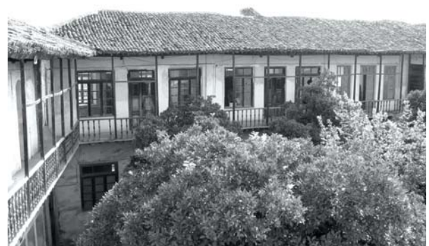
Fig. 6: A view of the northern front of first family courtyard before the restoration operation
