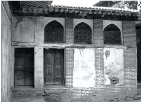
Fig. 11: Blocked openings in the first family courtyard and samples of existing and blocked herringbone windows
