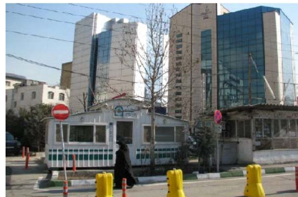
Fig. 2: A walkway with low level security (Chizar, northern corner of Neda Square, spring 2011)
