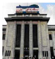
Fig. 6: Railway station Tehran
