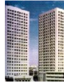
Fig. 11: Saman residential tower
