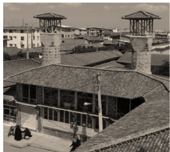
Fig.6: Gable Roofs in Panjshanbe-Bazaar Covered with Tiling
