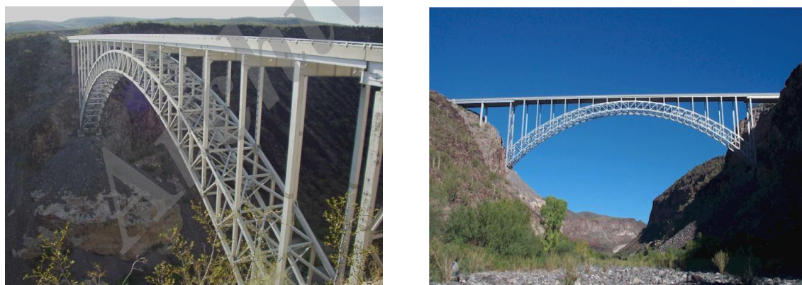
Figure 1. Burro Creek Bridge
