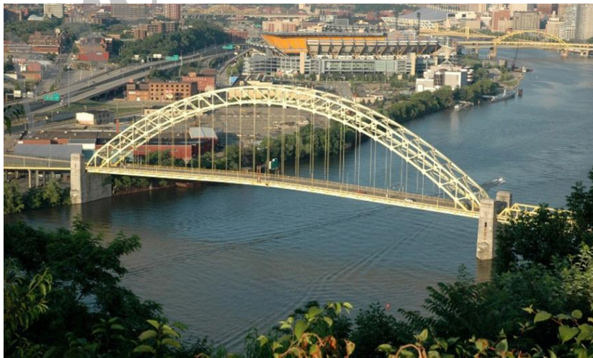
Figure 5. The West End-North Side Bridge
