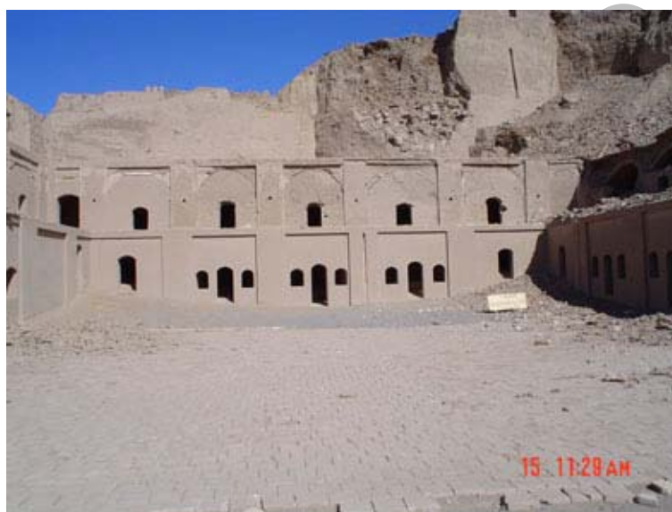
Figure 2. The east-west wall of the Military citadel in Arg-e-Bam.
