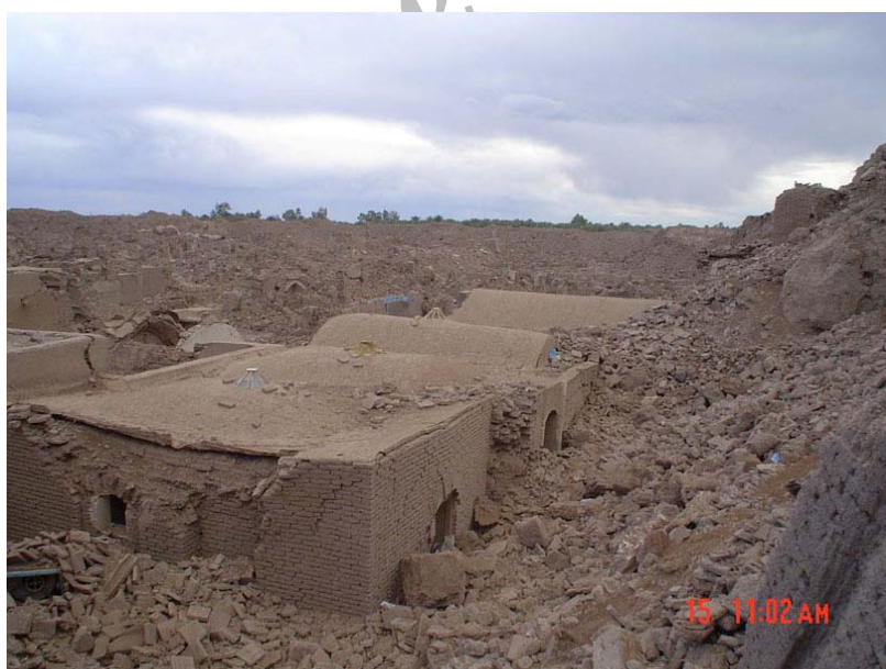
Figure 5. The two types of vaults that are commonly used in Bam, Tharbi and Kalil
