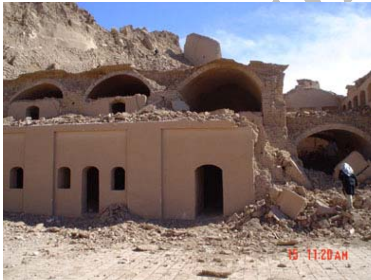
Figure 3. The north-south wall of the military citadel in Arg-e-Bam.
