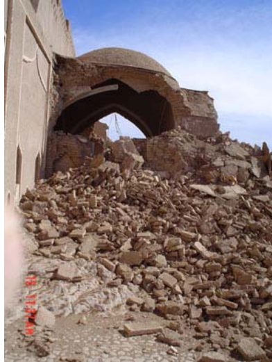
Figure 10. A dome supported by two walls and two arch panels.
