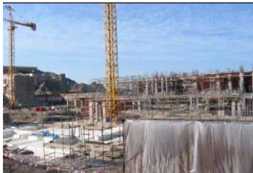
Figure 15. Overview of the construction site of a seaside Building Complex. Stainless steel reinforcement is used in the outer exposed structures from below ground water level up to level +5m. See Figure 16.
