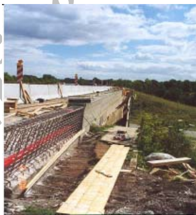
Figure 18. Replacing edge beams and parapets on Danish bridges and crash barriers on the motorways exposed to de-icing salt. SSR is introduced to avoid future repairs as well as avoiding the serious delays and inconveniences to the users, an issue becoming more and more in focus with the growing awareness of the costly societal consequences of such delays.
