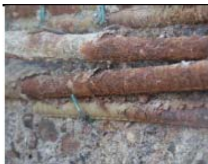
Figure 23. Details of the corroded epoxy coated reinforcement shown on Figure 21. The loose layer of epoxy on the corroding bar is clearly visible
