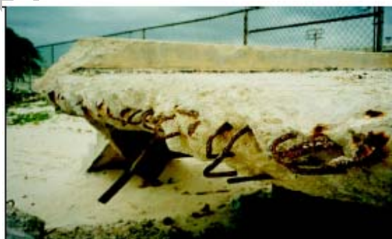
Figure 14. Close-up of the land based remaining parts of the “new” pier of which part of the remaining piles are shown in Figure 13. This pier was reinforced with ordinary black steel reinforcement and lasted only about 10 years.
