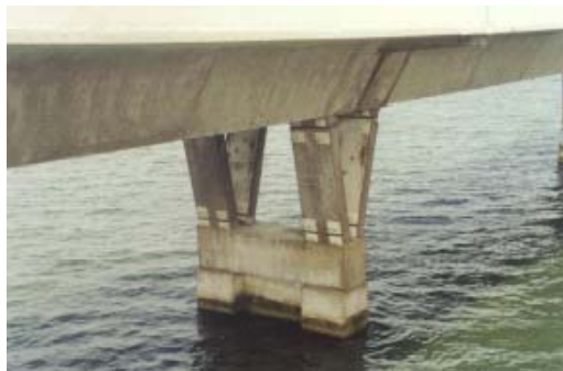
Figure 20. Bridge on the Florida Keys. Critical corrosion of epoxy coated reinforcement leading to splitting of the V formed supports now strengthened by prestressed bolts
