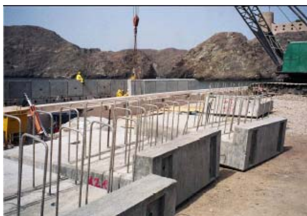
Figure 17. Stainless steel reinforcement used in the precast structural members to replace a corrosion damaged seawall protecting the existing important buildings and the new Building Complex (Figure 15) from the Gulf.
