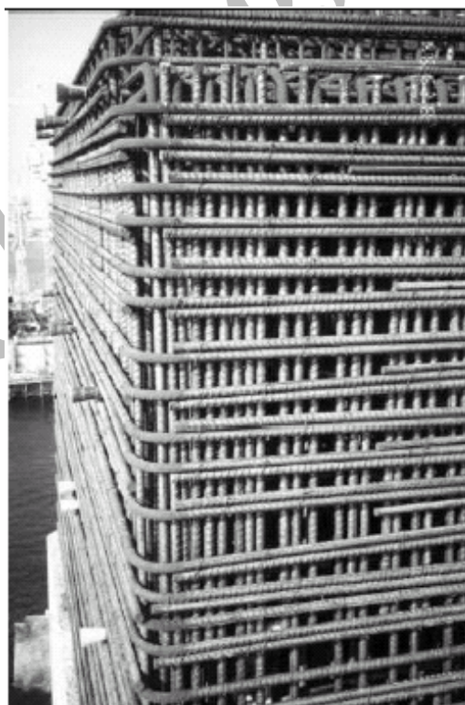
Figure 11. Example of reinforcement detailing which does not respect the need for reliable casting and compaction of concrete. Particularly the quality of the concrete "skin" (the cover) is in danger
