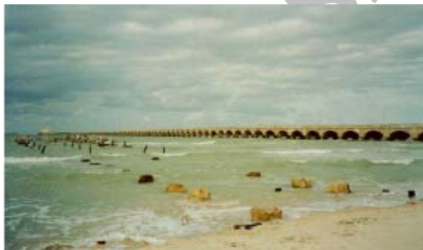
Figure 13. 65 year old stainless steel reinforced pier at Progreso in Mexico still fully intact without maintenance whereas the remains in the foreground is what is left of an only about 30 year old pier reinforced with ordinary black steel reinforcement, see Figure 14.
