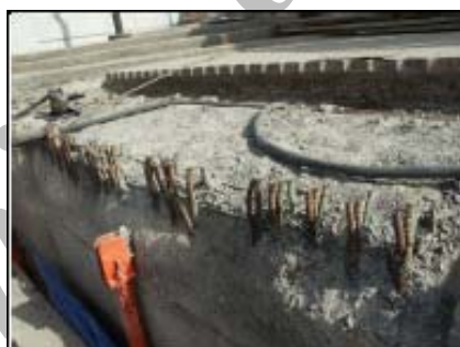
Figure 21. Seawall reinforced with epoxy coated reinforcement-heavily damaged by reinforcement corrosion after about 12 years
