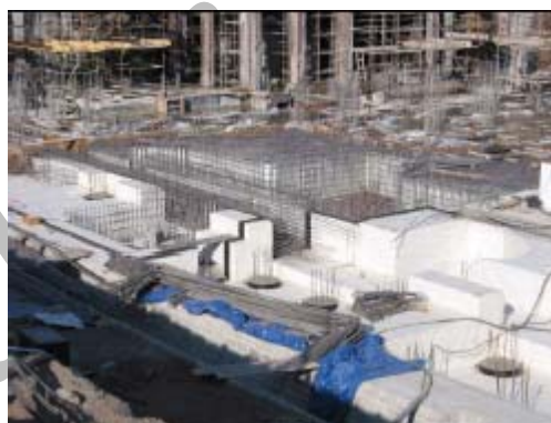
Figure 16. Detail from Figure 15. The remaining reinforcement is ordinary carbon steel. The design service life without corrosion damage is 50 years.
