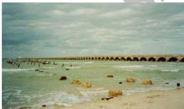
Figure 13. 65 year old stainless steel reinforced pier at Progreso in Mexico still fully intact without maintenance whereas the remains in the foreground is what is left of an only about 30 year old pier reinforced with ordinary black steel reinforcement, see Figure 14.
