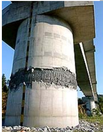
Figure 3. Severe but promptly repairable damage
