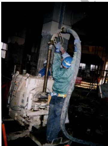
Figure 11. Compaction grouting in basement of existing building
