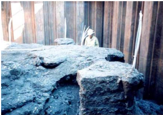
Figure 26. Excavation of subsoil grouted by seeping of silicate liquid.
