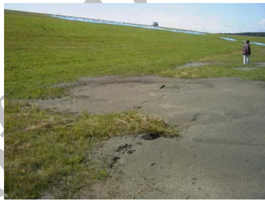
Figure 8. Minor liquefaction near dike of Tokachi river in 2004. earthquake
