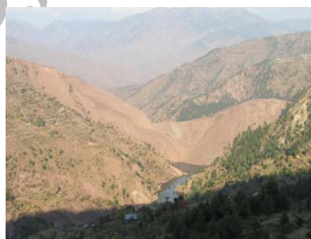
Figure 2. Slope failure and natural dam near Chakar in Pakistan during the Kashmir earthquake in 2005
