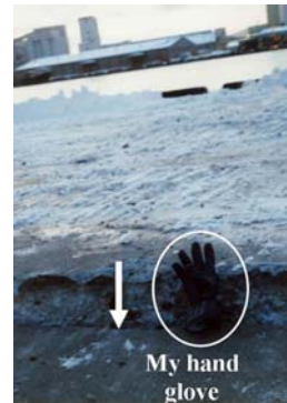
Figure 10. Minor subsidence in Kushiro Harbor in 1993 in spite of heavy seismic shaking
