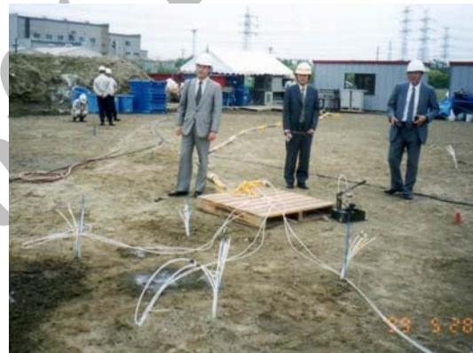
Figure 25. Seeping of silicate liquid into sandy ground
