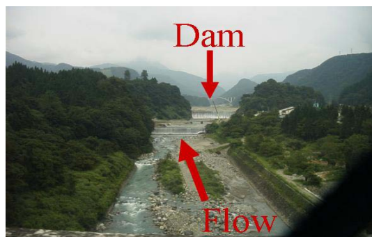
Figure 19. Erosion control dam to stop migration of debris to downstream area (mitigation on path).
