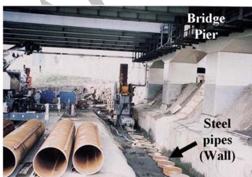
Figure 13. Sheet pile wall as mitigation
