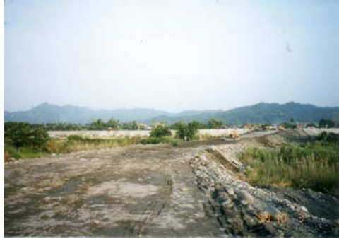
Figure 3. Quick construction of detour road after 1999 ChiChi earthquake in Taiwan
