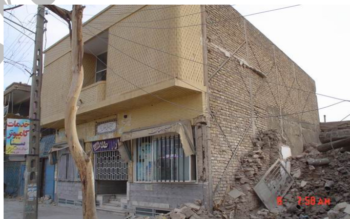
Figure 8. Steel building with good performance during the Bam 26.12.2003 earthquake
