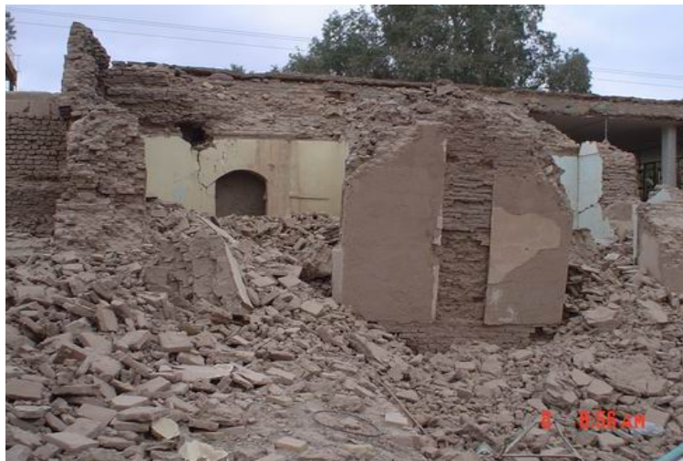
Figure 4. Heavy walls-thickness of wall in some adobe houses is around 1 m
