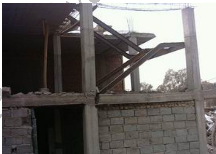
Figure 12. Use of steel stair in a reinforced concrete structure
