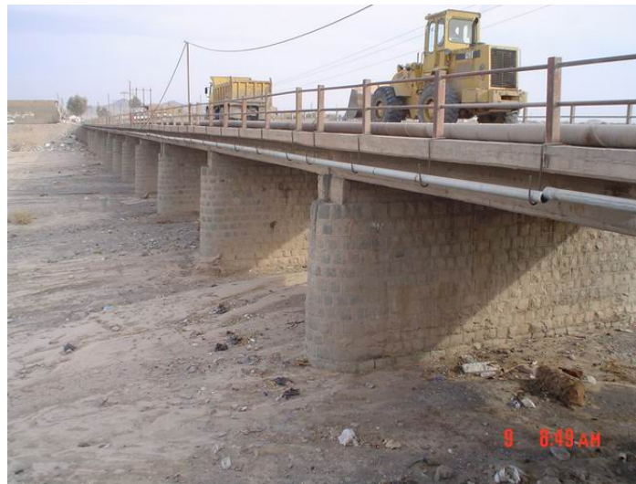
Figure 16. General view of the multi spans Reinforced Concrete Bridge after the earthquake which is in good condition and of course under service.
