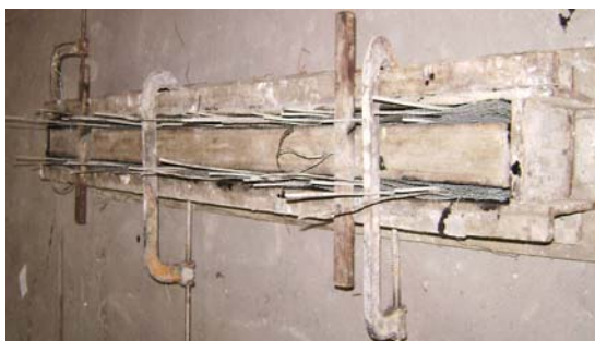
Figure 2. Placement of wire mesh with solid mould for pouring mortar.
