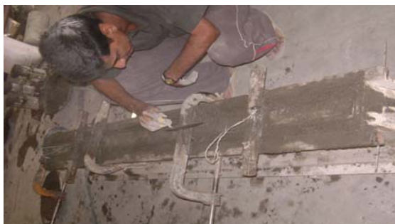
Figure 3. Mortar is filled through wire mesh leaving the core portion
