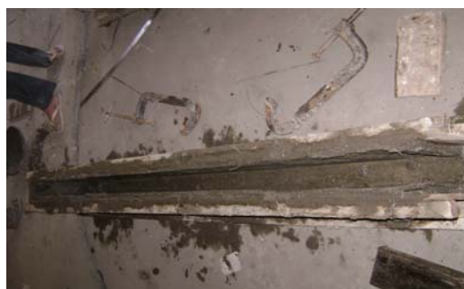
Figure 4. Ferrocement shell in the mould ready for casting of core concrete
