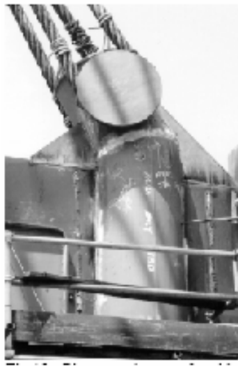
Figure 5. Pipe trunnions for side block lift
