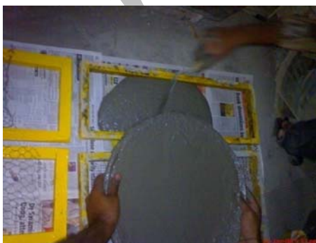
Figure 3(a). Placing of mortar into moulds
