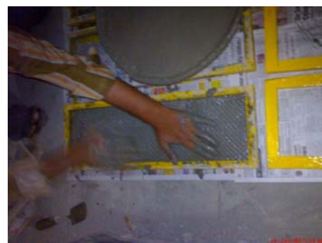
Figure 3(b). Placing of mesh
