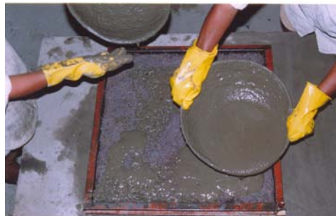
Figure 2. Casting of SIFCON slabs
