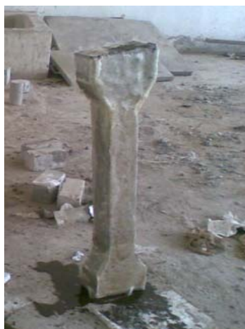
Figure 6. Wrapped short columns
