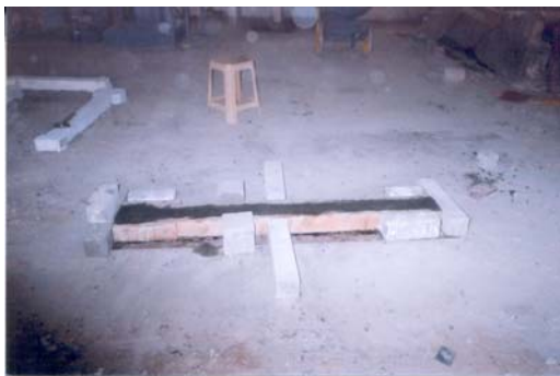
Figure 3. Casting of test specimen
