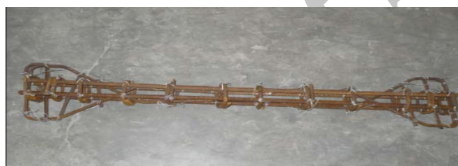
Figure 2. Reinforcement cage for short column
