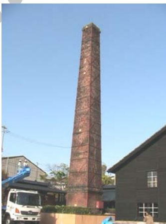
Figure 5. Appearance of the chimney
