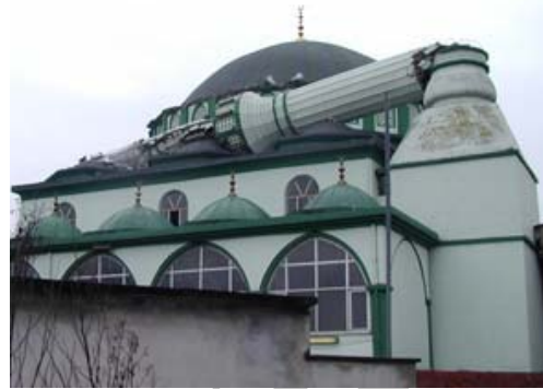
Figure 2. Collapse of minarets due to failures near the bottom of the cylinders
