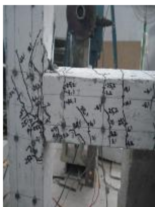
Figure 9. Failed monolithic specimen
