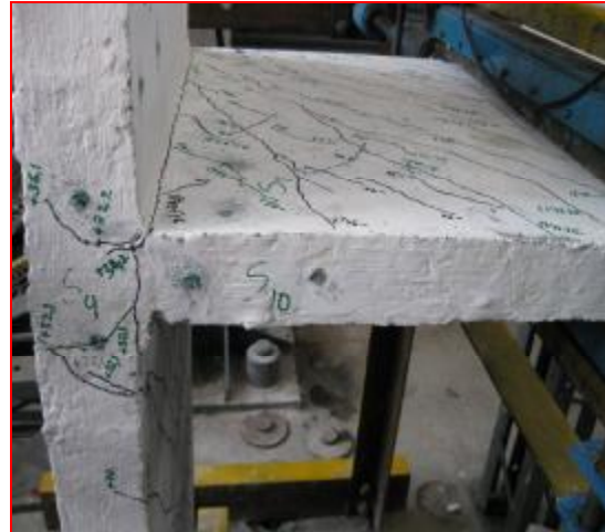
Figure 7. Cracks in Type 2 specimen
