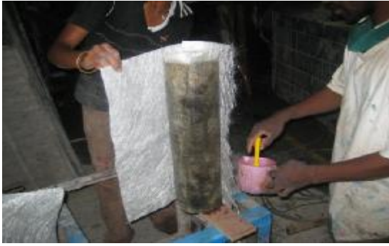
Figure 4. Wrapping under progress
