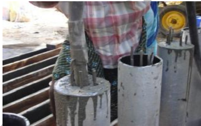
Figure 3. Casting under progress
