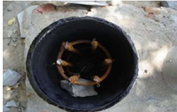
Figure 2. Reinforcement cage with cover block
