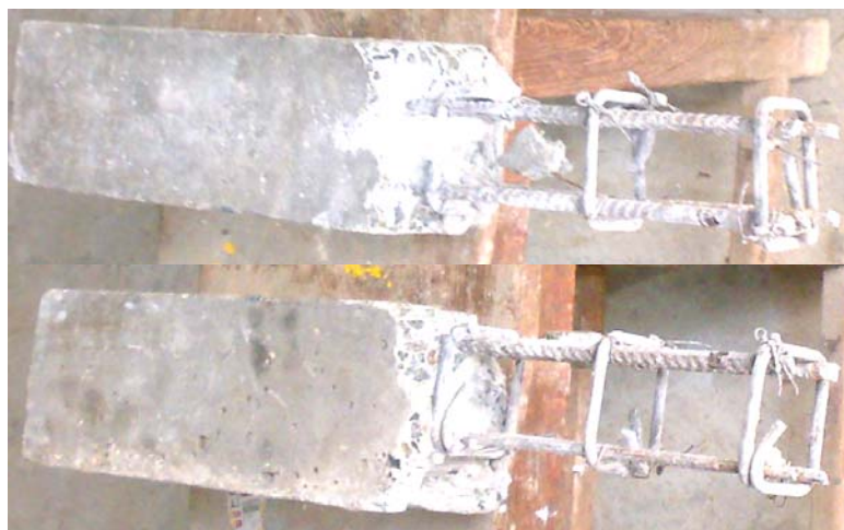
Figure 8. Top-uncorroded rod in specimen 'A' Bottom-uncorroded rod in specimen 'B'
