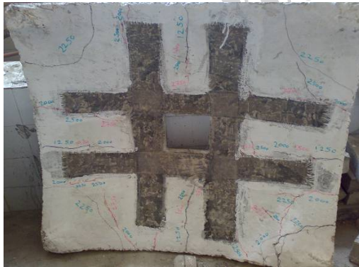
Figure 22. Crack pattern of shell "SOG1" strengthened by using 2 layers GFRP (Type 1). [Failure load = 3500 kg]
