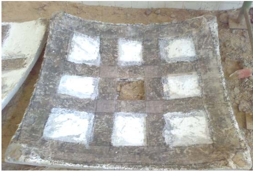
Figure 9. Repaired shell "ROG2" by using 2-layers of GFRP wrap (Type 2).
