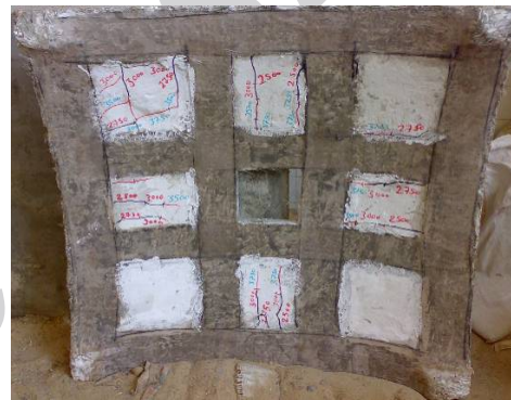
Figure 27. Crack pattern of shell "ROG2" repaired by using 2 layers GFRP (Type 2). [Failure load = 3750 kg]
