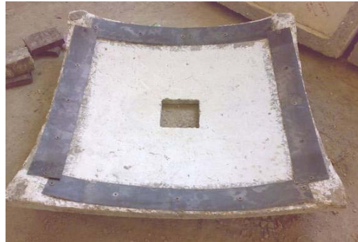
Figure 10. Repaired shell "ROS" by using steel strip.
