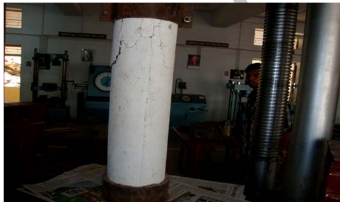
Figure 5. Failure pattern of SFRC column
