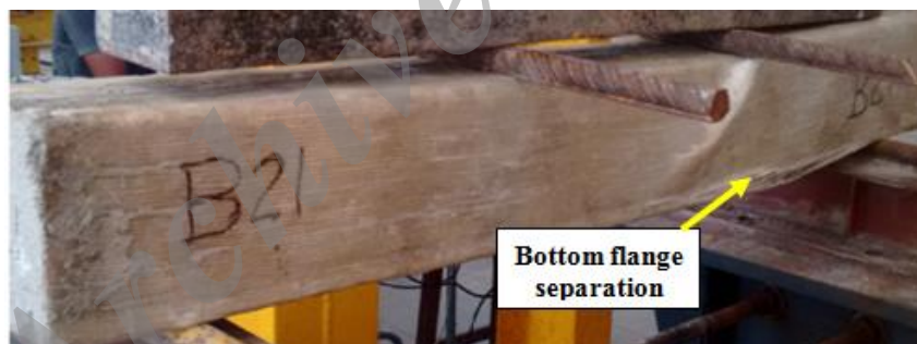
Figure 13. NSC infilled WR GFRP tubular beams (R2W)
