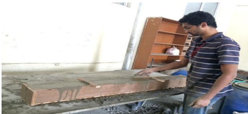
Figure 4. Casting of beams
