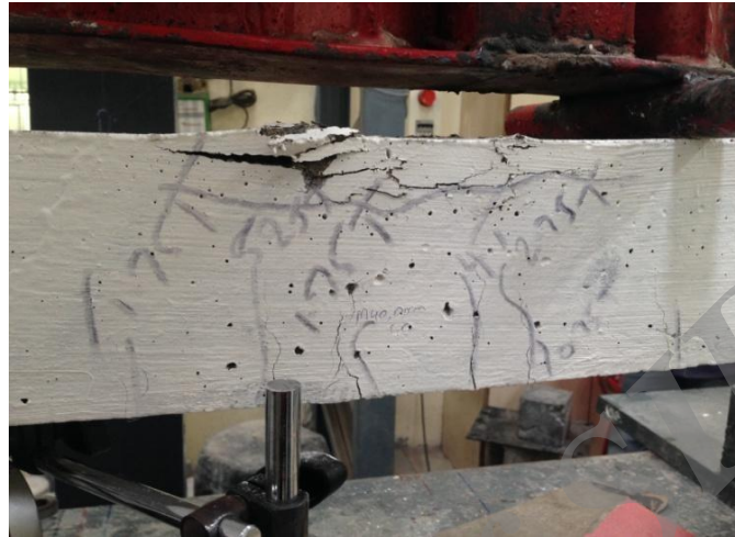
Figure 7. Crack pattern of beam
