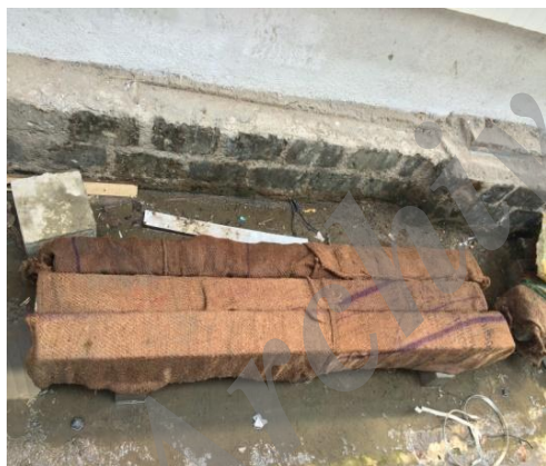
Figure 5. Curing of beams
