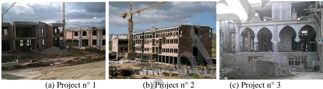
Figure 1. Overall view of the projects
