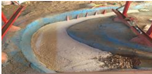
Fig. 3- a view of installed triangular vanes installed
