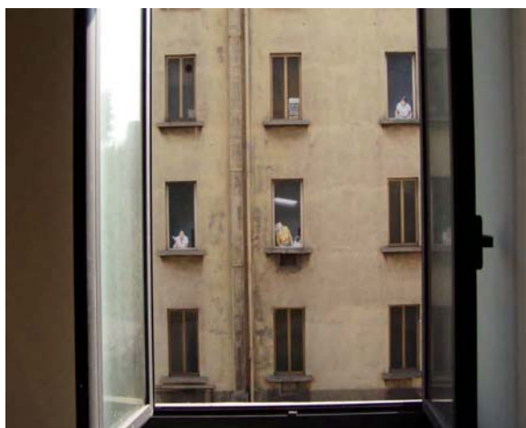
Fig.1. Absence of citizens Piombino-Tuscany Proximity of the industrial environment Inhabitants and residents are “absent” or, quite paradoxically, show up only when depicted on the façades of the buildings
