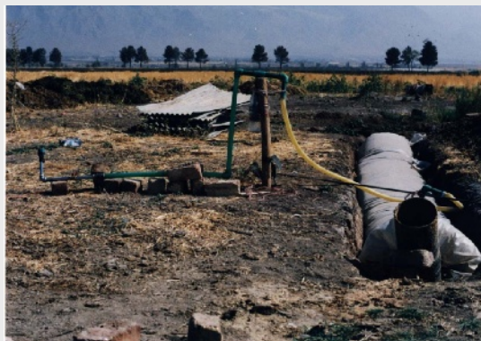
Figure 2. Installed polyethylene biogas plant.
