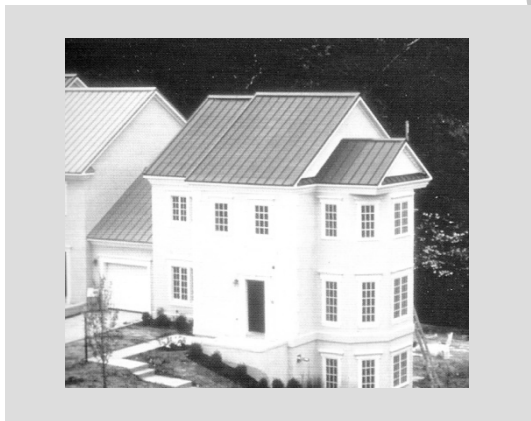
Figure 1. PV on a dwelling in Maryland, USA (Prasad and Snow, 2005).
