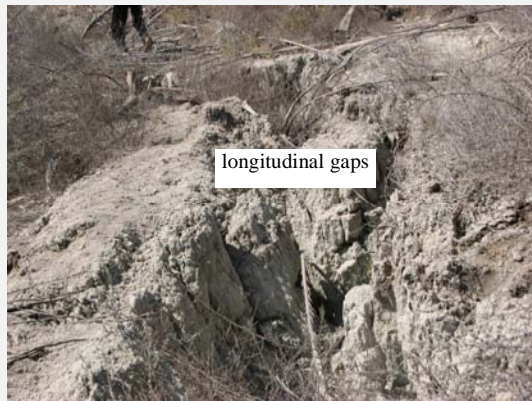
Figure 16. Existed longitudinal gaps in both sides of subsidence.
