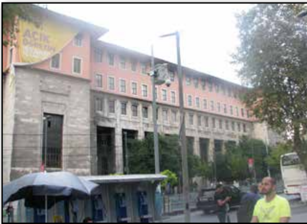
Fig.16. College of science and literature, artwork of Sedad Hakki Eldem, Istanbul, 1942. Photo: Naser Hassanpour, 2014.
