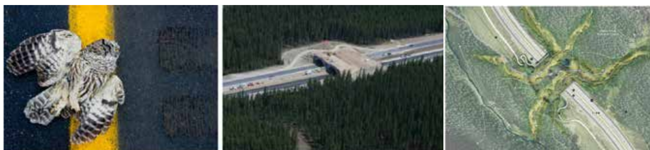
Fig. 3. Examples of eco-paths crossing a highway. Using barriers and technological materials to inform the species to prevent accidents or provide certain types of conditions for their migration, and restoration of damaged circulation of dynamic ecological phenomena such as water circulation are some types which including news specialized topics to focus on. Source: OREG, 2010.
