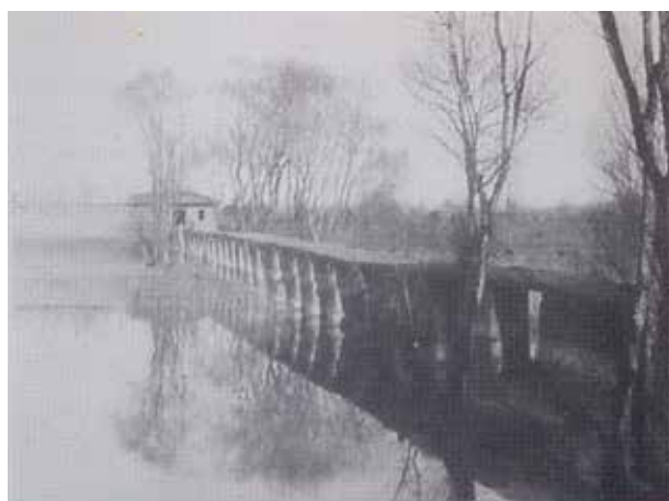
Fig. 5. Wooden bridge of Bahrol-eram in 1891; composed of 29 stone pillars and a wooden floor, which provided the only access to the lake, located along the street leading to Sabze Meidan. Source: Elahi, 2006: 19.
