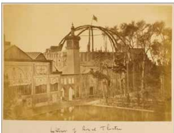
Fig. 1. Outer area of Tekyeh Dowlat, special system for building roof, photo: Smithsonian Collections Online (Courtesy of Smithsonian). Source: Sevruguin, 1933.
