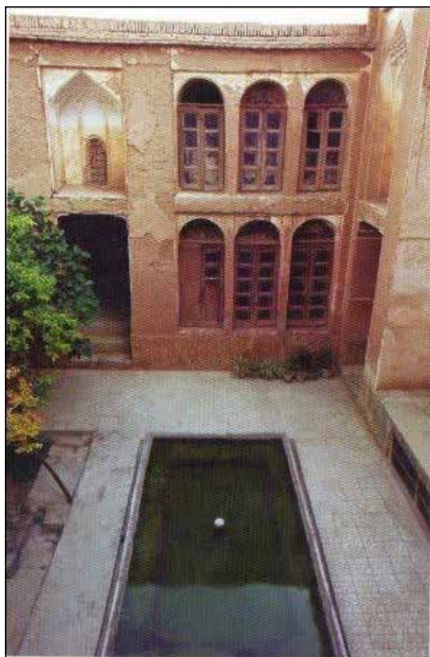
Fig. 2. Tehrani's house before repurposing.
