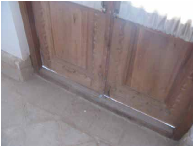
Fig. 7. The gap between the door and frame in "2- door" room of Oloomi's house causing infiltration. Source: author.
