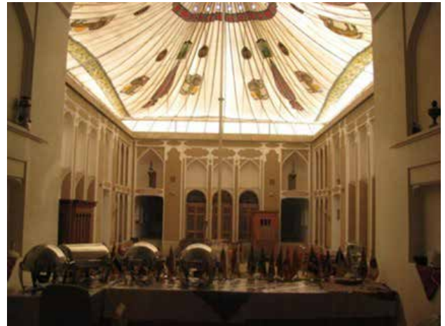
Figure 9. Raising permanent canvas structure on the courtyard and preventing direct solar absorption. Source: author.
