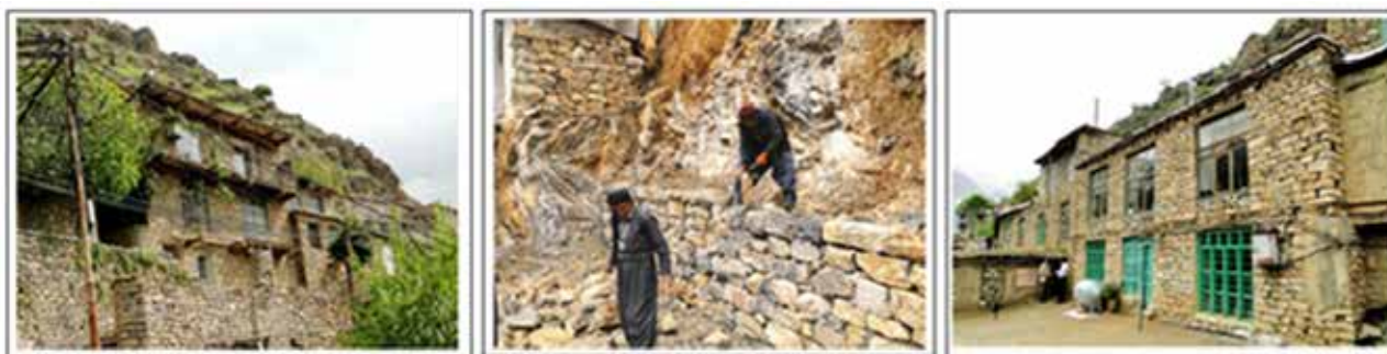
Fig. 4. Stone, wood and soil are the main materials of construction on Hawraman. Source: authors.
