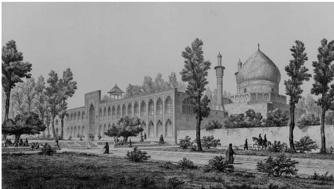
Fig. 2. Khiâbân-Chaharbaq of Isfahan (School of Shah Sultan Hossein's mother) in middle of 13th century AH. Landscaping of the street (khiâbân) is affected by Iranian garden concept. Drawn by Pascal Coste (Architect) who visited Iran in 1840 along with Eugene Flandin (painter). Source: Shirazian, 2018.
