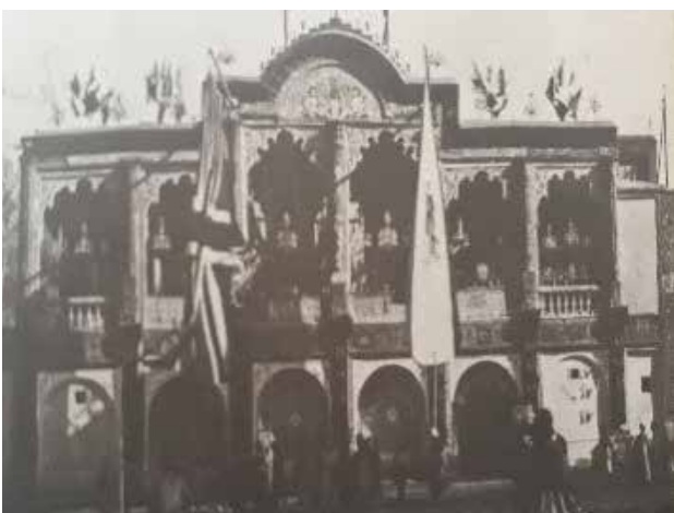
Fig.2 The image on the top is the transom of the Shah Bank, Tehran (Source: Cultural Research Archive in Soltanzadeh, 2005). In down: The building is characterized by Roman semicircular arches, pediments and Corinthian capitals, and the image on the left is a building in Almasia (Source: Soltanzadeh, 2005): It is characterized by a crown pediment.
