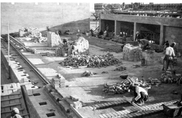
Fig.1. Stages of construction of Karaj smelter factory. Source: www.holzmann.fh-potsdam.de
