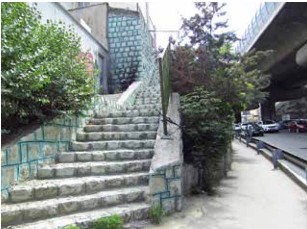
Fig. 7. The non-inclusive stair structure of the sidewalk neglecting the rights of disabled people. Source: authors' archive.
