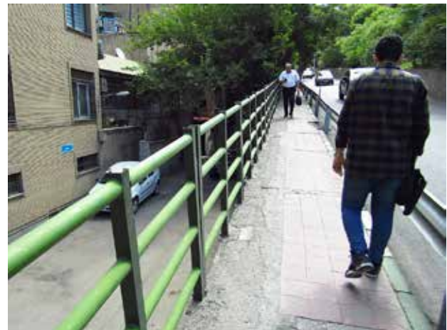
Fig. 6. A non-inclusive sidewalk with an extreme slope, low width, and inappropriate pavement. Source: authors' archive.
