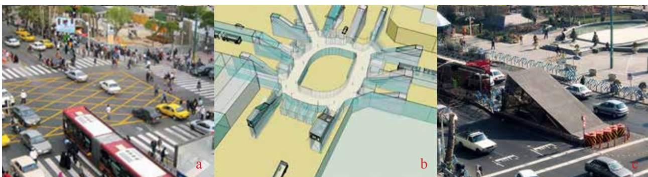
Fig. 4. Vali-e Asr Crossroad: (a) The situation of crossroad before the construction of the underpass; (b) 3D graphic design of the proposed pedestrian underpass; (c) One of the entrances of the underpass towards the underground. Source: www.isna.ir and www.meidaan.com.
