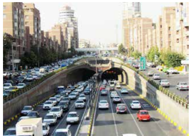
Fig. 3. Navvab highway as a completely totalitarian design. Source: authors' archive.
